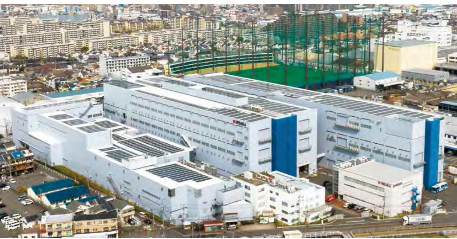
HISAKA WORKS / Konoike Plant
